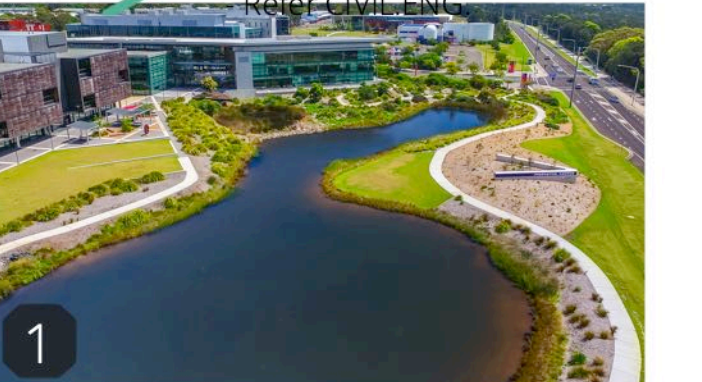
1 The Existing Lake/Onsite detention collects stormwater runoff from across the Innovation Campus.
