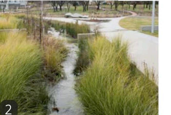
2 The Bioswale / Basin receives site runoff and filters/purifies water before being released to existing lake/onsite detention and Fairy Creek
